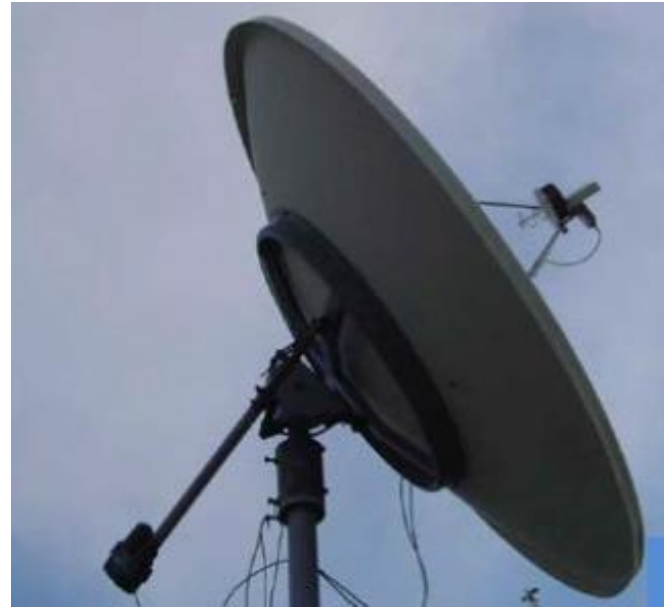
IAASARS/NOA MSG SEVIRI Acquisition station DVB-S2
