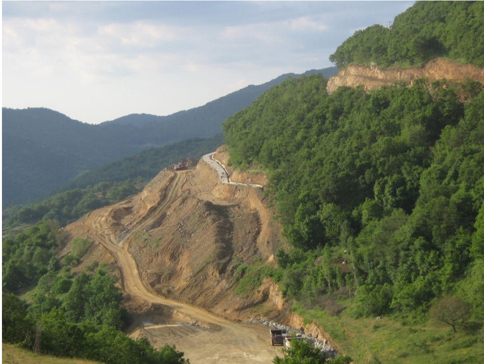
Fig. 83 Photo of cut slope O21 during excavation (part A, Efraimidis, 2009)
